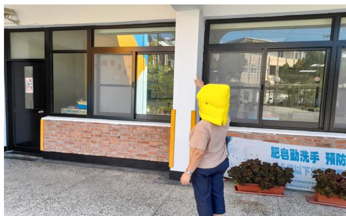
說明—檢查建築物牆壁有無龜裂
