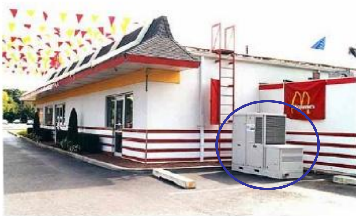
McDonald's restaurant in North Babylon (NY) partially powered by a fuel cell (Source: LIPA)
